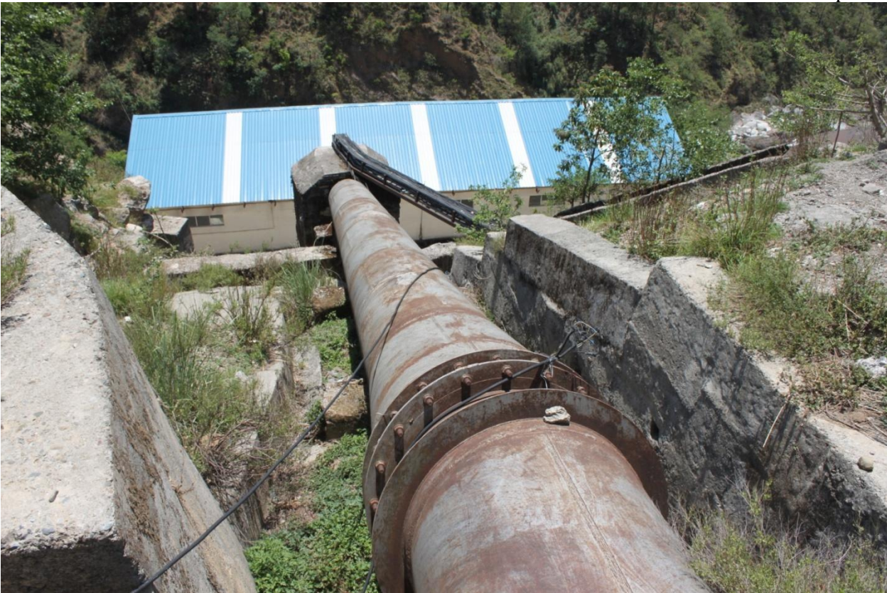
Picture 2: A tunnel diverting river towards power house
